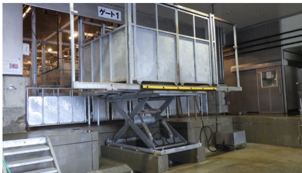
*Photo: Example of Facility C
