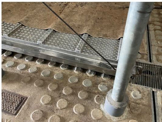
*Photograph: Example of Facility A
